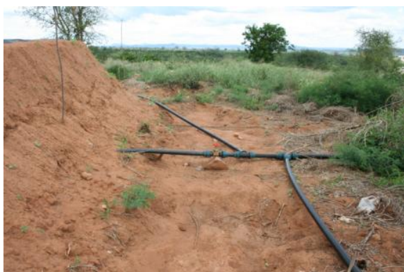
Figure 31: Network of pipes for water division
